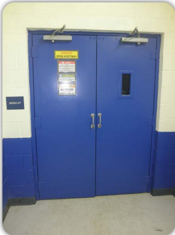
Double swing fire-rated doors
